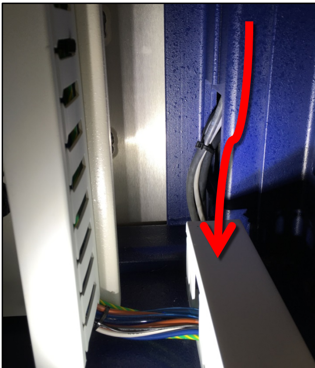
Pull cables through bottom corner/chassis opening.
