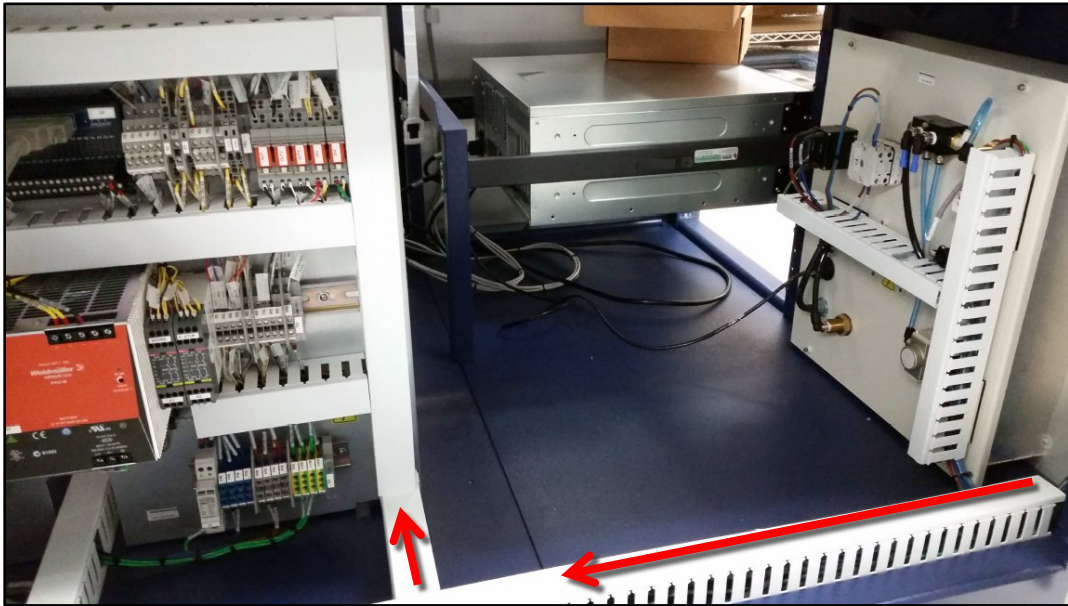
Route cables toward ePlate #2.
